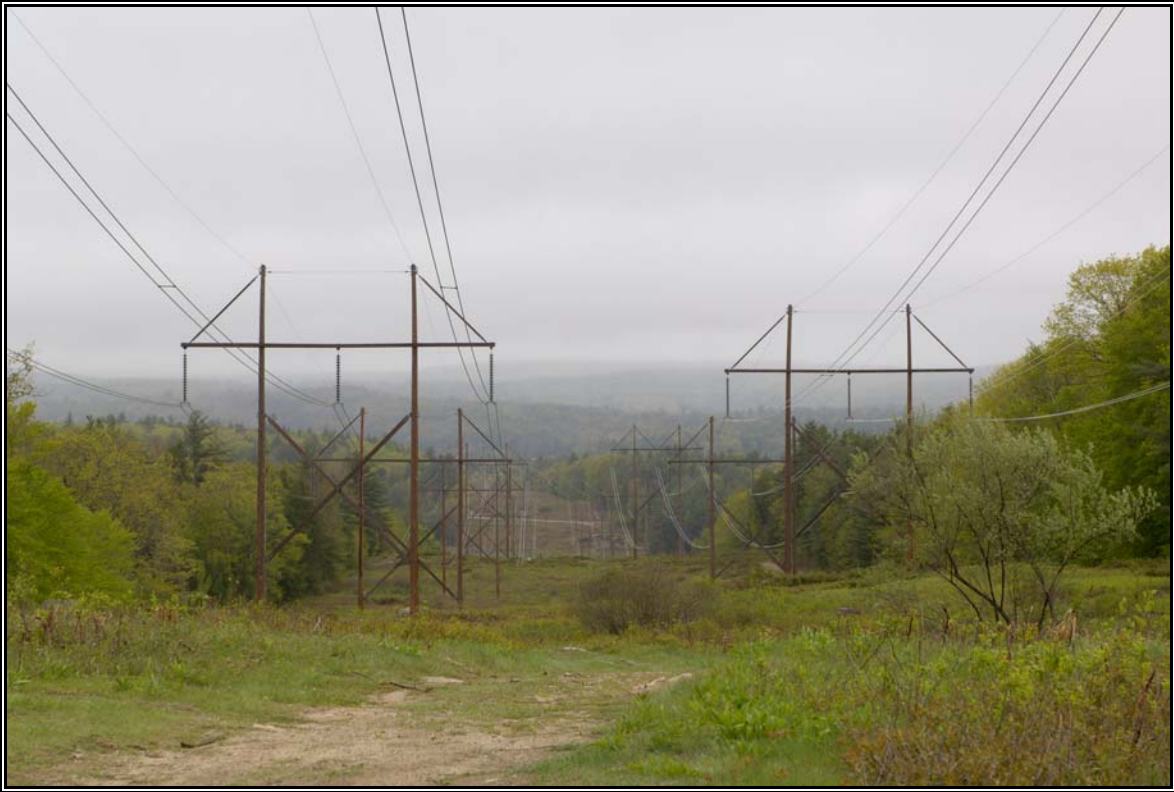
HVAC Power Line Corridor in Deerfield
